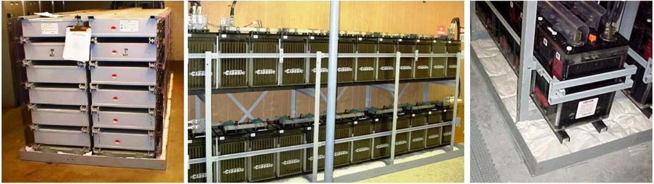
Spill control systems are rapidly becoming standard equipment in facilities containing stationary battery systems. Batteries contain sulfuric acid and an unintentional release could cause a number of potential hazards including:
